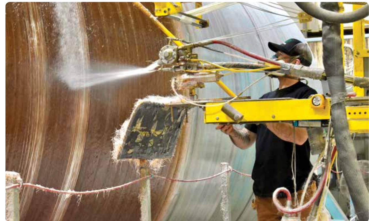
Chop-Hoop Filament Winding storage tank.
